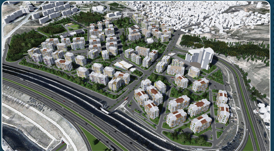
Uzundere Urban Transformation Area
